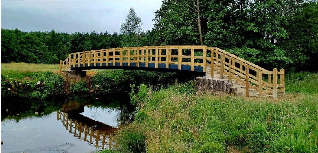
Figure 13 Plump Wood Footbridge, Nunnington
